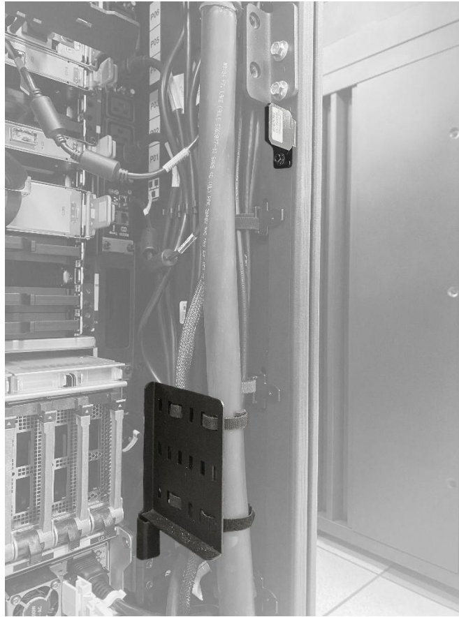
Figure 7: Use Hook-and-Loop to Retain Line Cord and Keep Away from Latch
