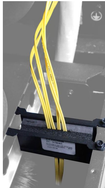
Figure 39: Strain Relief Clamp
