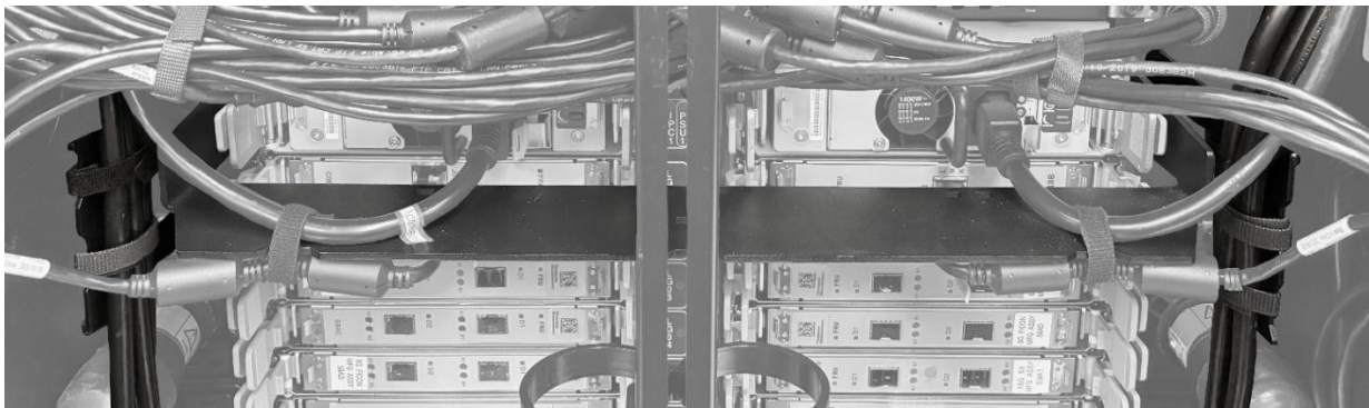
Figure 23: Vertical Cable Management Brackets
