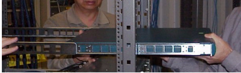
Figure 2-6: Sliding the Switch Into the Rack
