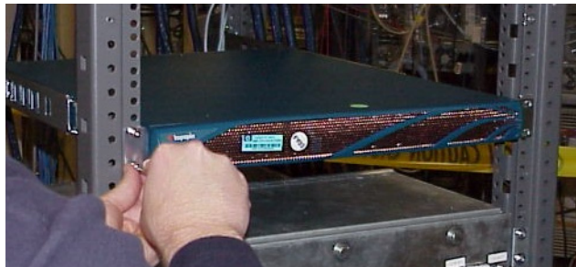
Figure 2-7: Secure switch with screws through the front of the rack
