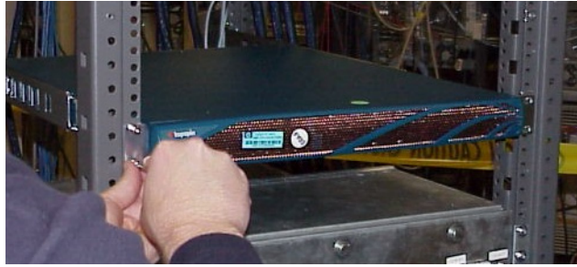
Figure 2-10: Secure the Switch Through the Front Rack Rail
