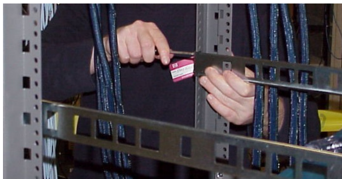
Figure 2-5: Secure Rail Bracket to Rack with Screws
