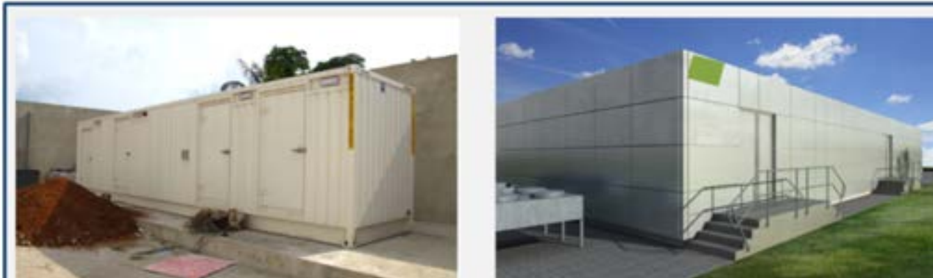
Figure 3. Choose a standard ISO shipping container in 20 or 40 foot lengths, or prefabricated modules that can be assembled into modular data centre buildings.
